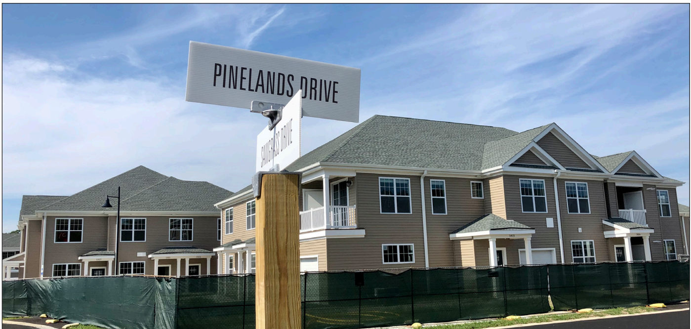
This 636-unit planned development in Hamilton Township, Atlantic County required the use of 45.75 PDCs.
